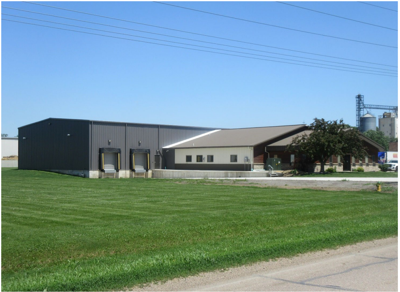
Warehouse addition – Dubak Electrical – Sheldon
