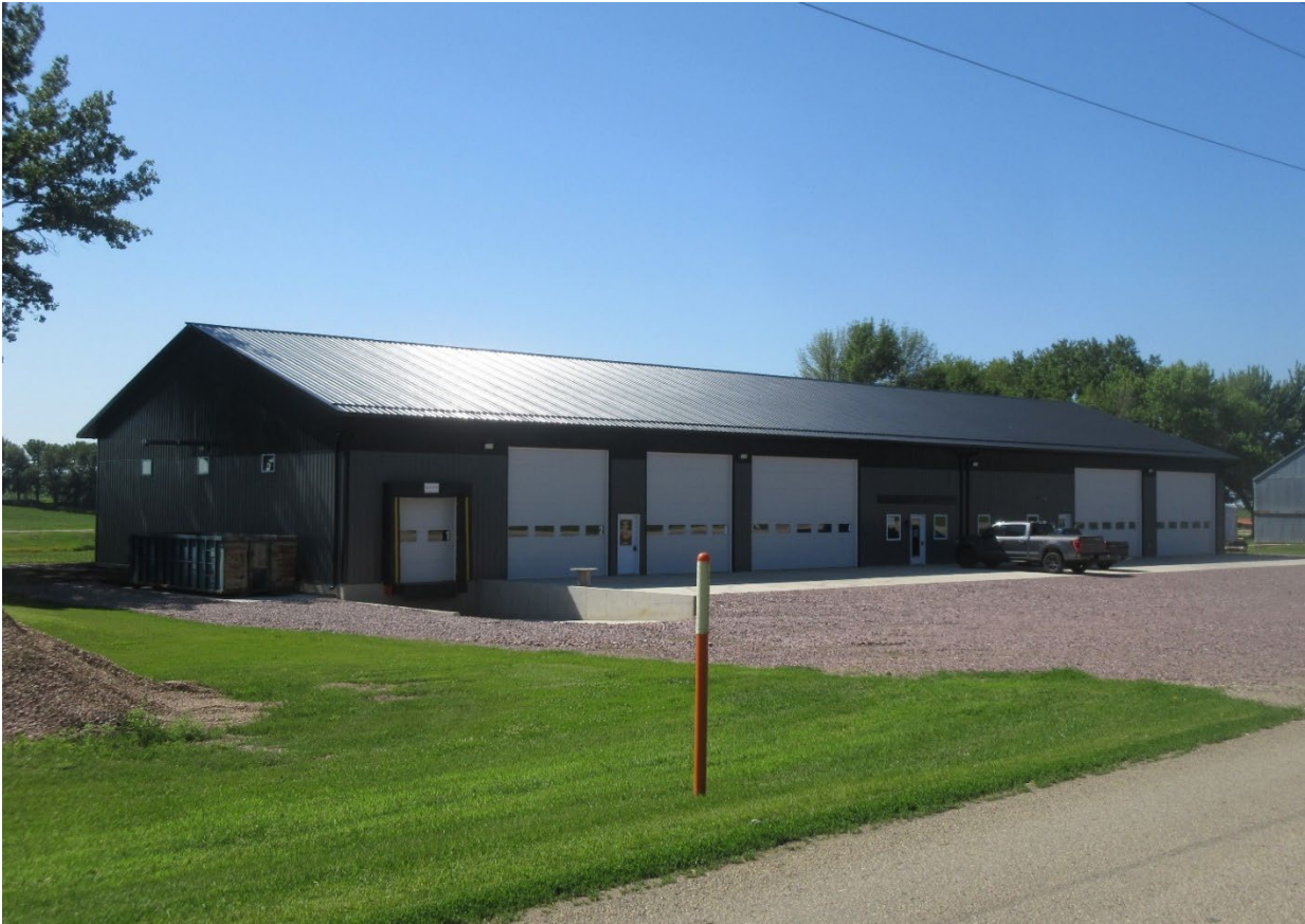
New shop for SRC Overhead Doors – Maurice
