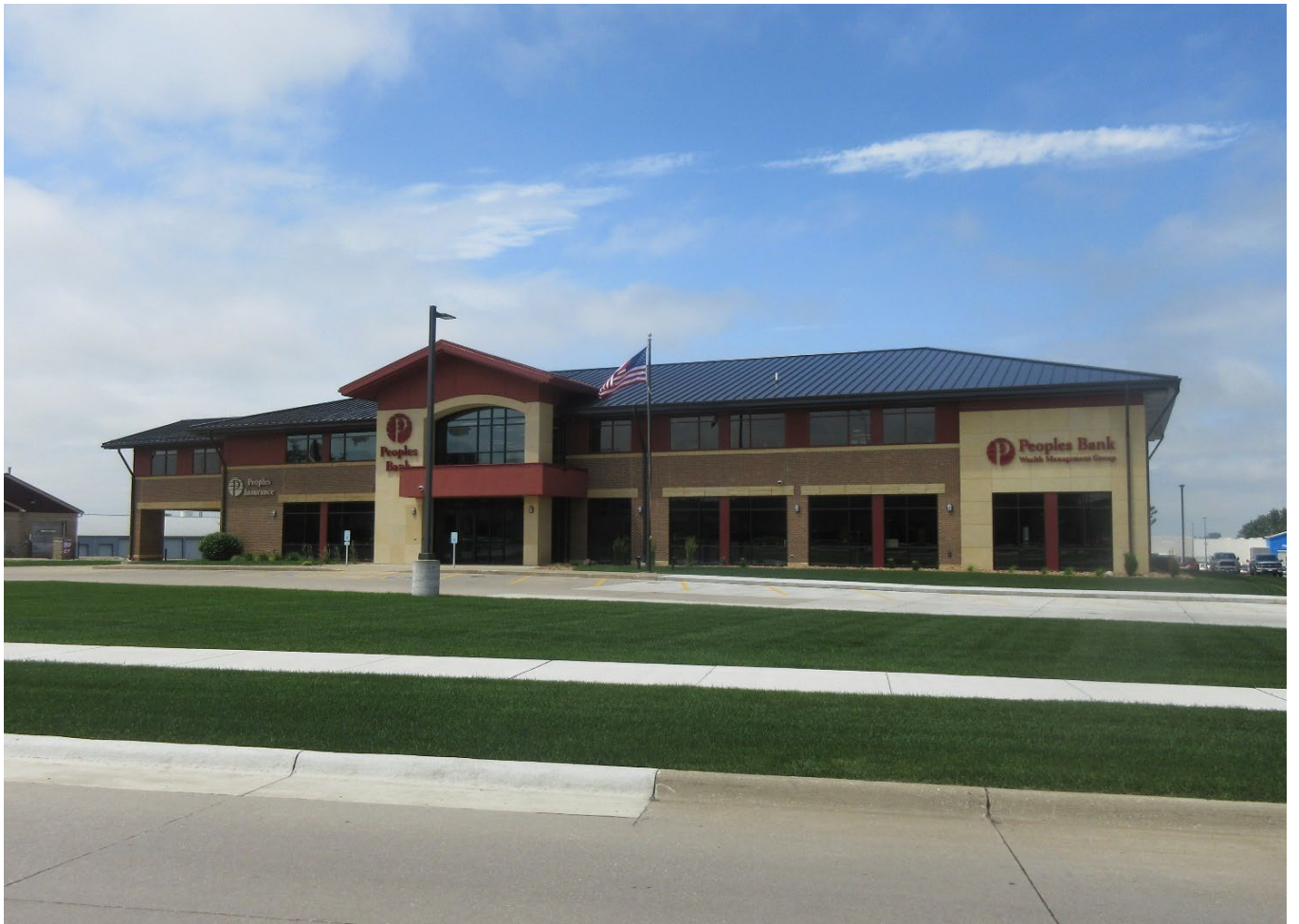
Addition – Peoples Bank – Sioux Center
