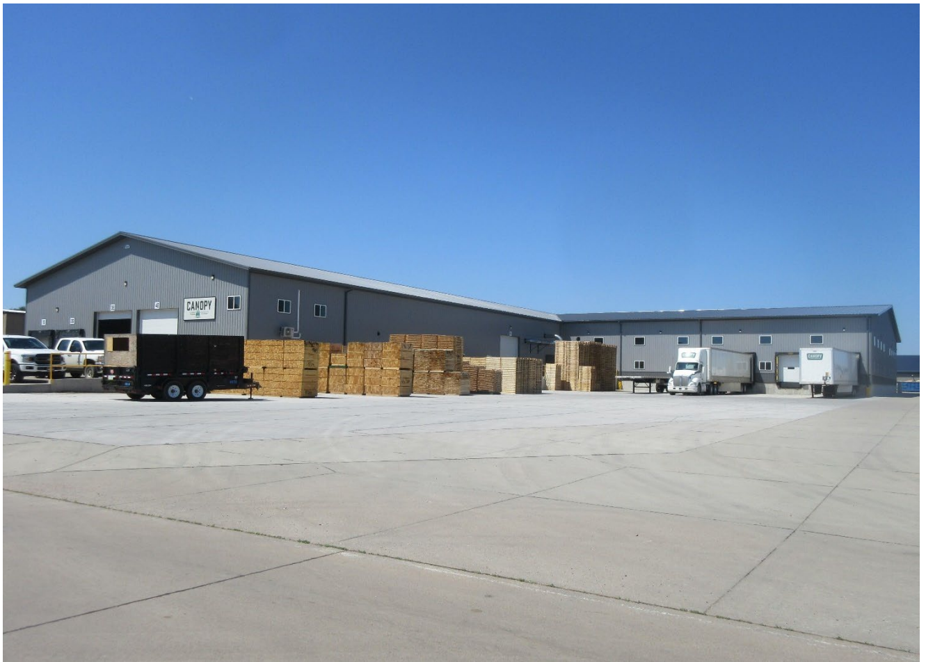
Addition on Canopy Lumber Products – Rock Valley
