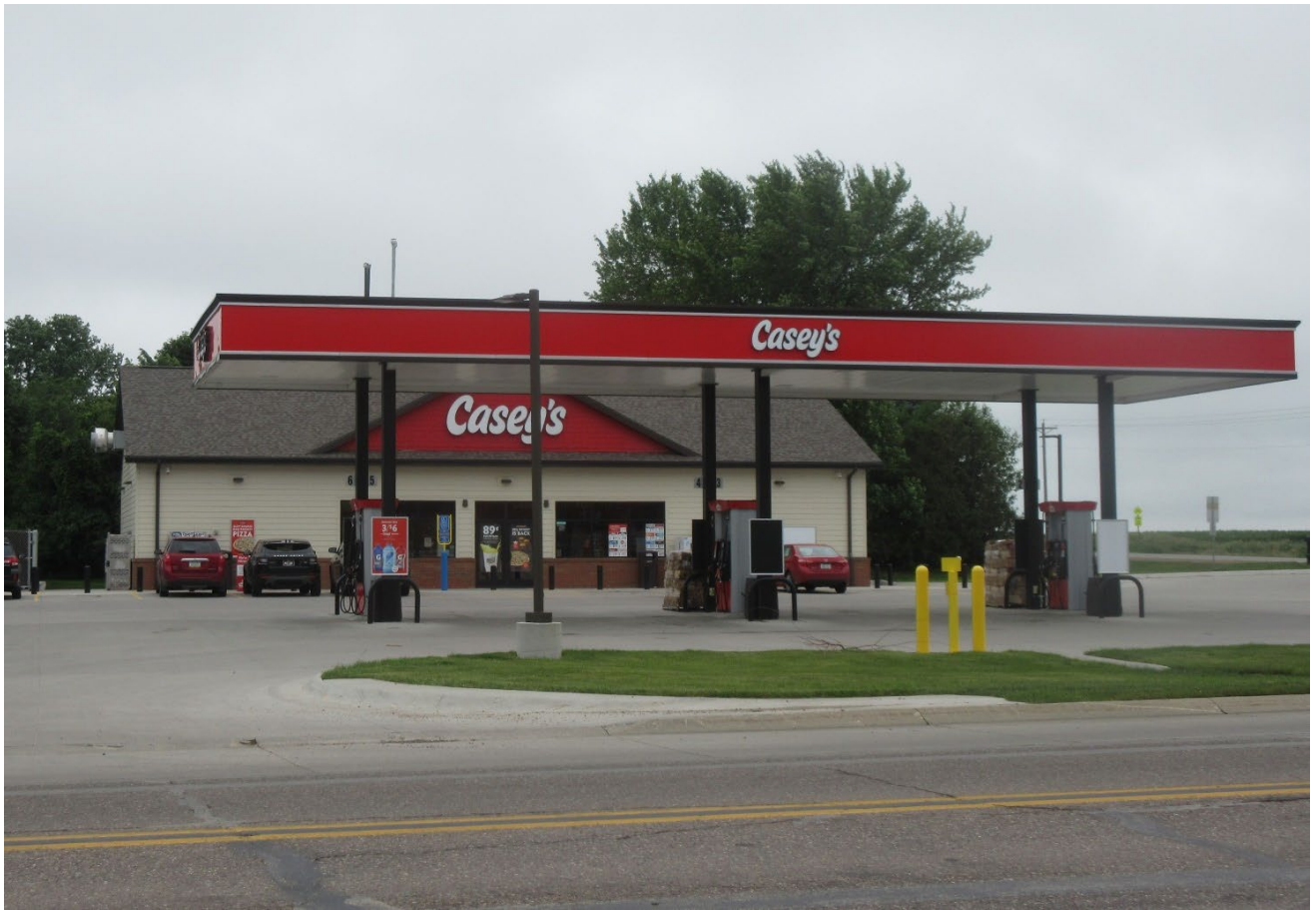
Replacement Caseys after fire – Hull
