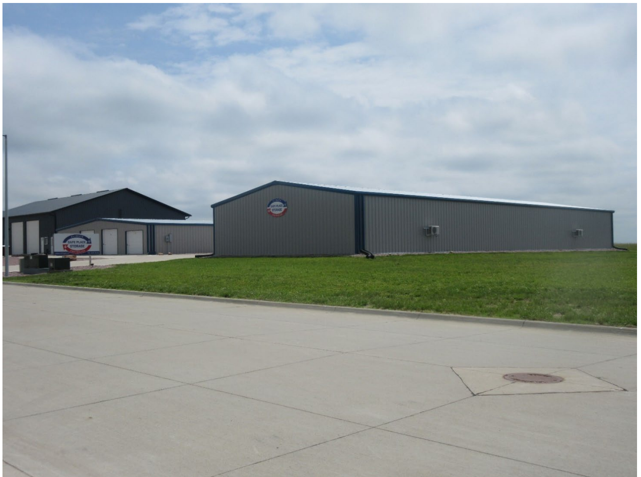
Expansion of climate control storage – Orange City
