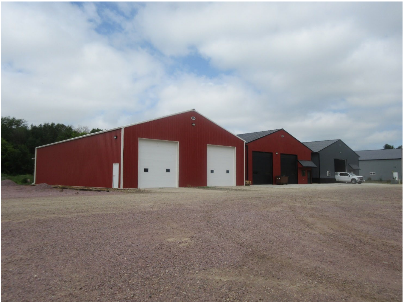
Commercial Warehouses – Alton
